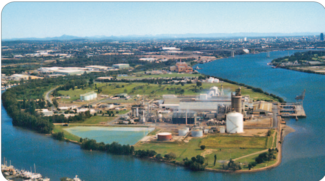
The Gibson Island facility. An HSEC highlight during the year was Reset 07, the major maintenance project which involved 1059 workers and 286,000 man-hours with only one injury requiring medical treatment.
